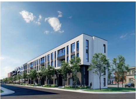
Requalification des ateliers Castelnau, Montréal © Provencherroy
