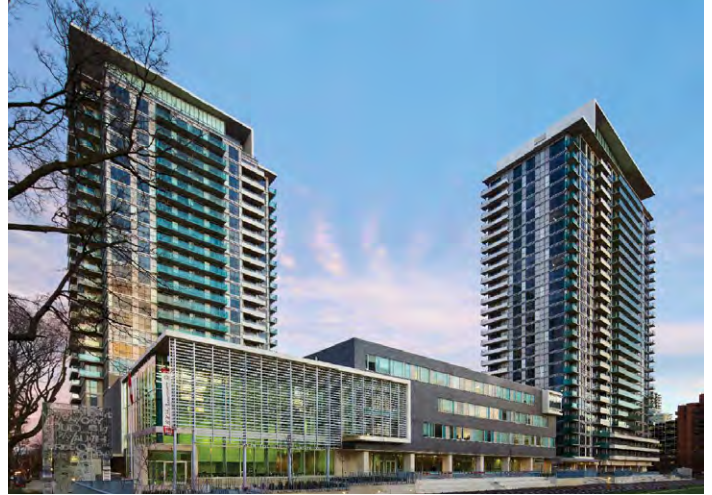
The North Toronto Collegiate Institute is integrated into the base of two residential towers. School amenities, including a theatre, classrooms and sports fields, are available to the community outside of school hours.
