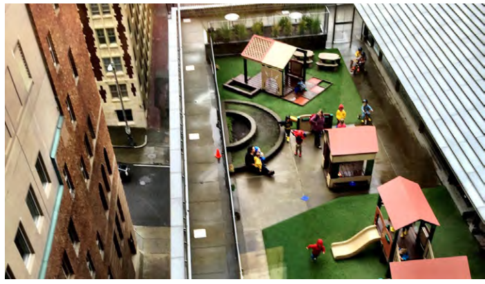
A roof top amenity playground in Seattle, uses turf grass as a surfacing material which functions as a green roof and provides a flexible play surface.
