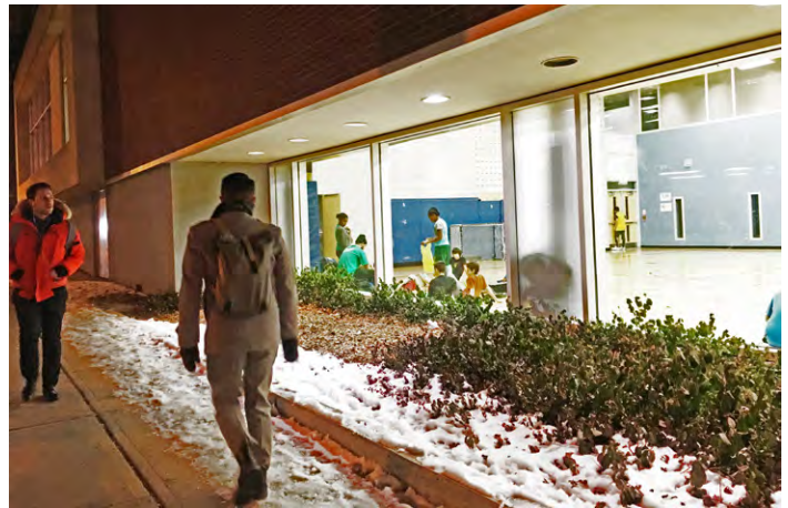
The active elevations at-grade at the Wellesley Community Centre in Toronto animate the public realm throughout the dark winter months.
