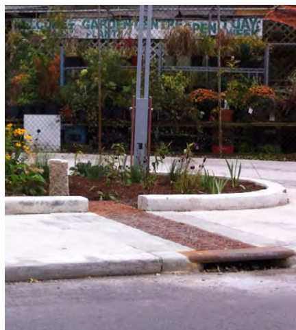
Fairford Avenue Parkette in Toronto was created by reducing the adjacent vehicular traffic lanes. The new parkette captures storm water runoff from the adjacent street, and provides furniture for resting while providing children access to nature. The storm water inlets are designed to be visible, to provide a learning opportunity.
