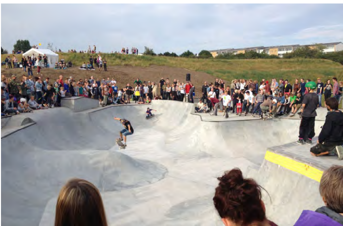
This skateboard park in Roskilde, Denmark functions as a floodwater drainage tool: the basin stores water when it rains and skaters can use the space when it's dry. The basin raises awareness about the need for storm water management.
