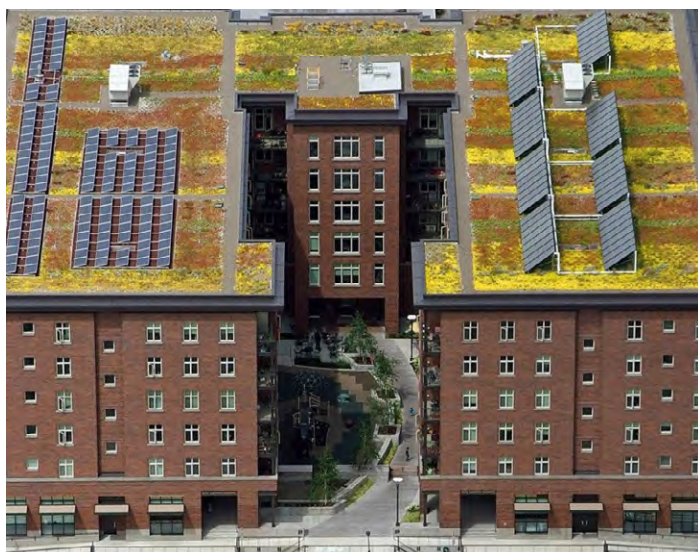
The "C" shaped Ramona building in Portland frames the central courtyard to create a safe, intimate open space which is visible from the street. Children playing in the courtyard can be supervised by the units overlooking this space.
