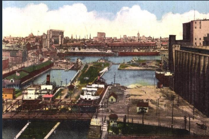
Pont tournant Black's Bridge
