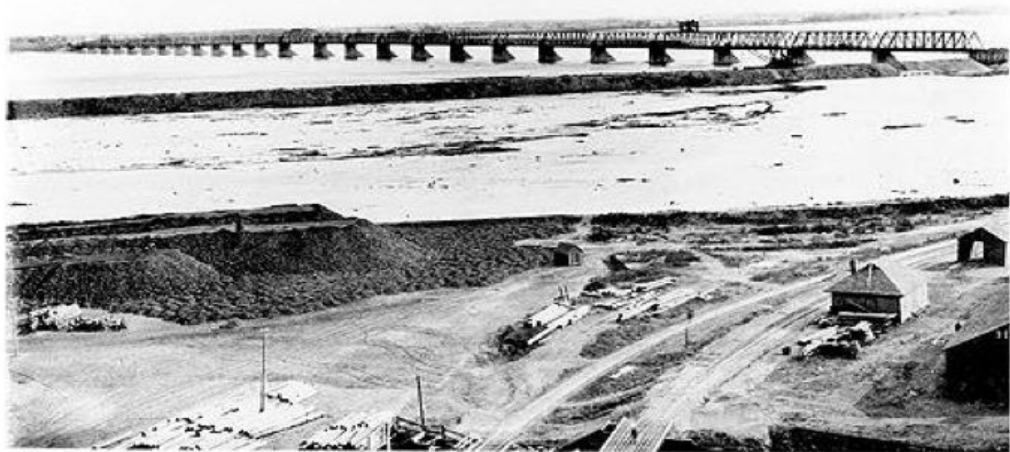
VICTORIA BRIDGE, G. T. R., IRON WORK 6502 FEET INCLUDING APPROACHES 914 FEET.
